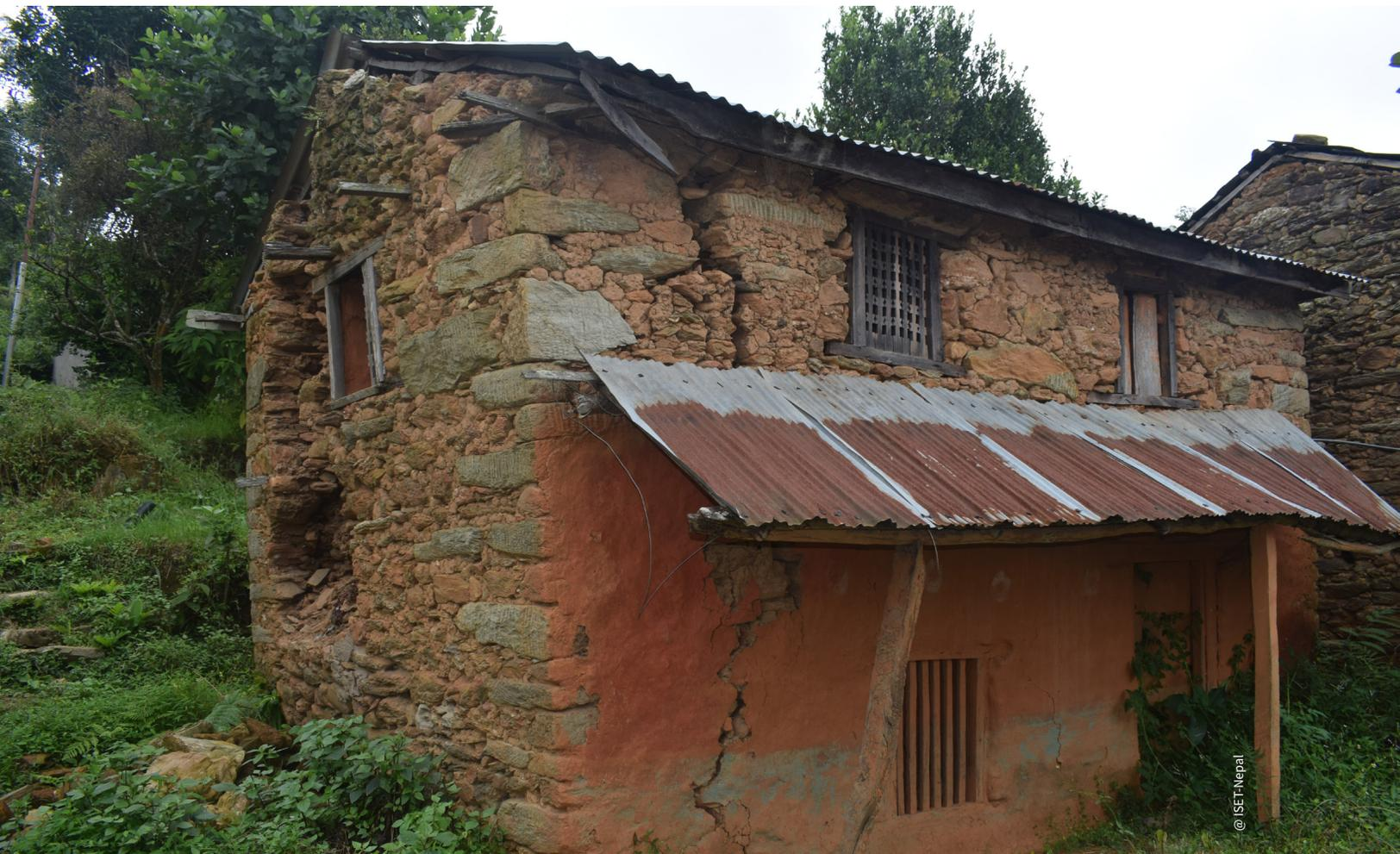
*Earthquake damaged rural house built in stone masonry in mud mortar, Nareshwar-3*
